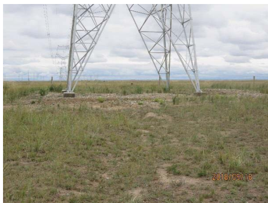
5#碎石压盖及施工场地恢复植被
