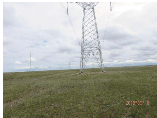
4#碎石压盖及施工场地恢复植被
