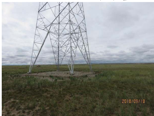
12#碎石压盖及施工场地恢复植被
