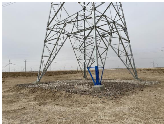
97#塔基区碎石压盖
