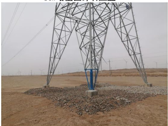
91#塔基区碎石压盖
